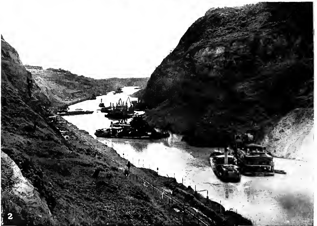
1. Looking south past Cucaracha slide, December 9, 1913. 2. Nine days later, looking north.
