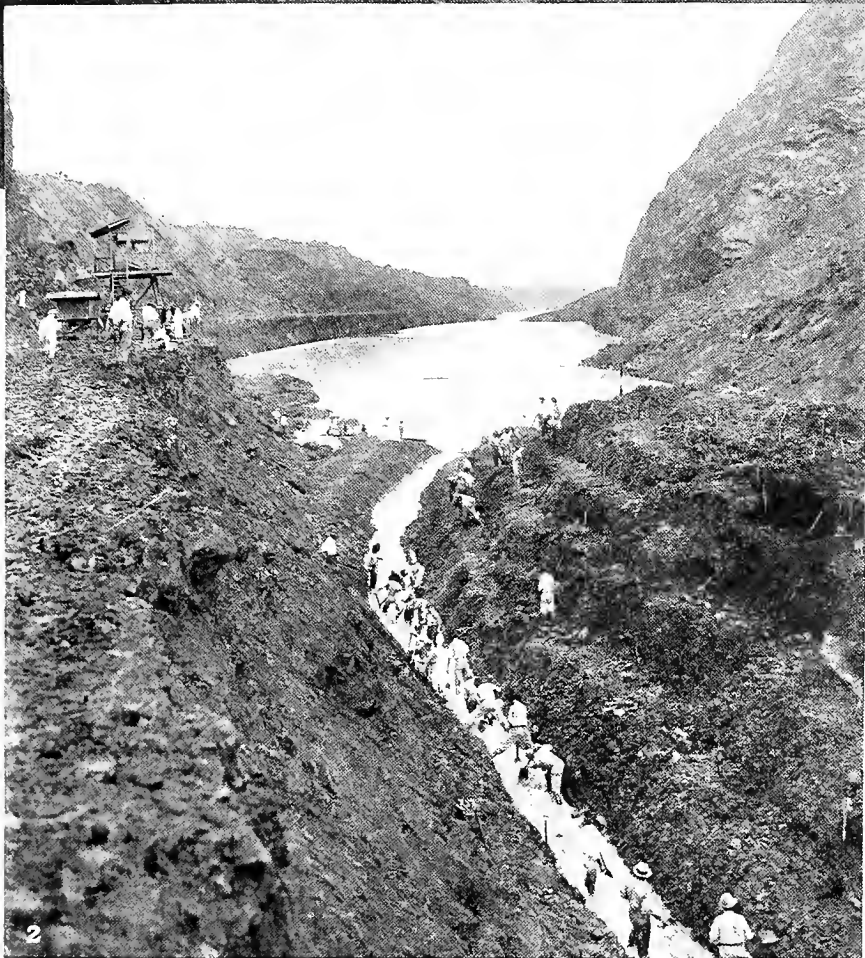
1. How Cucaracha slide came down many times a year and bottled up the south end of Culebra Cut. 2. Laborers trying to lead a stream of Gatun Lake water through the slide and down to Pedro Miguel.
